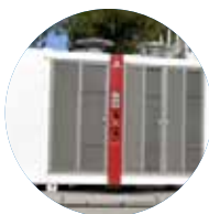
Backup fuel cell generator at the Atomic Energy Commission (Paris Saclay)
